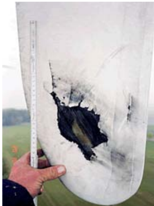
Example of blade damaged by lightning. (Photo by ARGE WEA, Austria)
